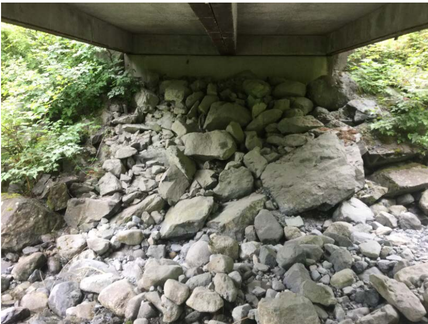
Right Bank Abutment when facing downstream
