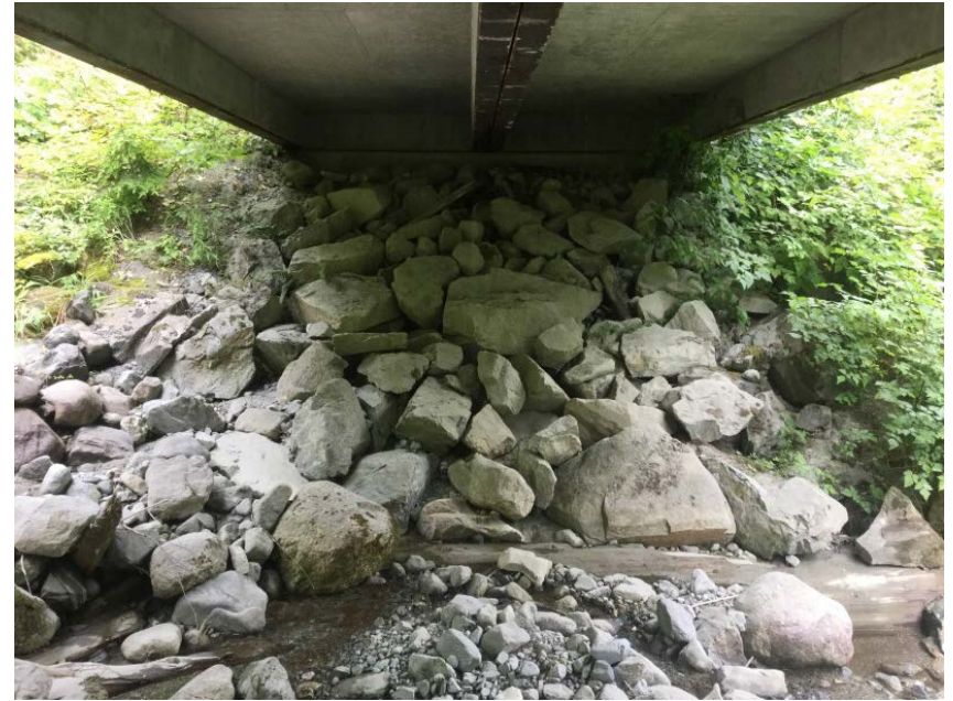
Left Bank Abutment when facing downstream
