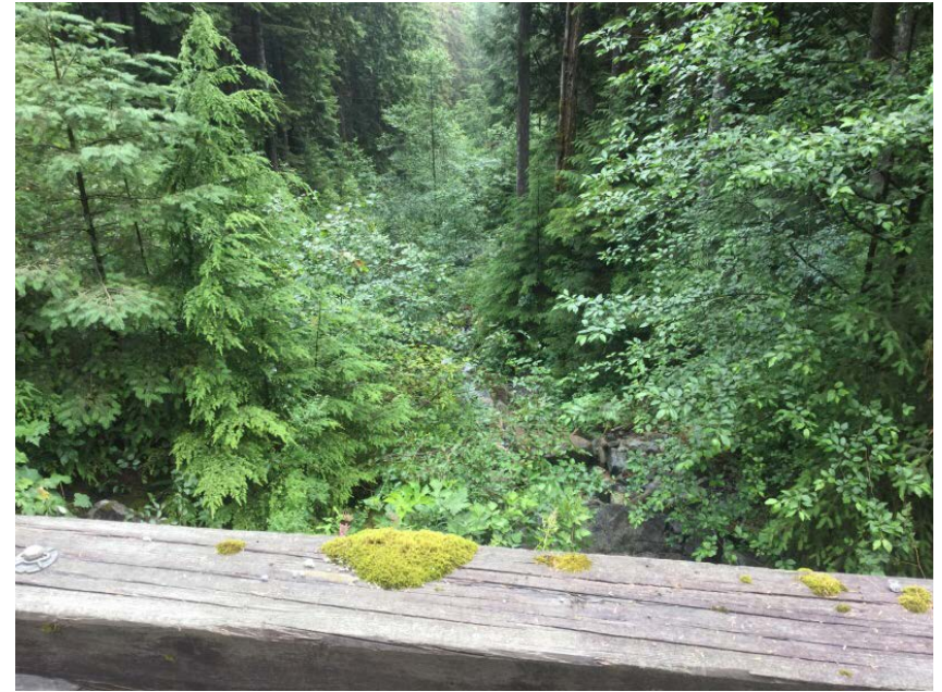
Looking downstream from deck
