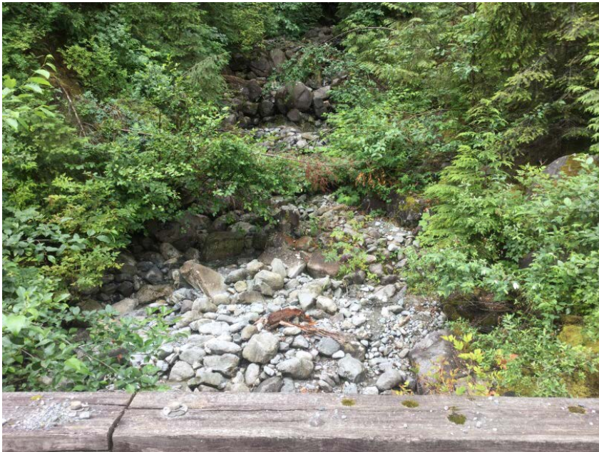
Looking upstream from deck
